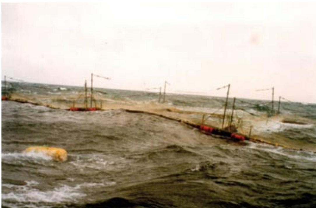
■ Figure 2.2 Rubber cage system flexing with waves at site in Sicily
