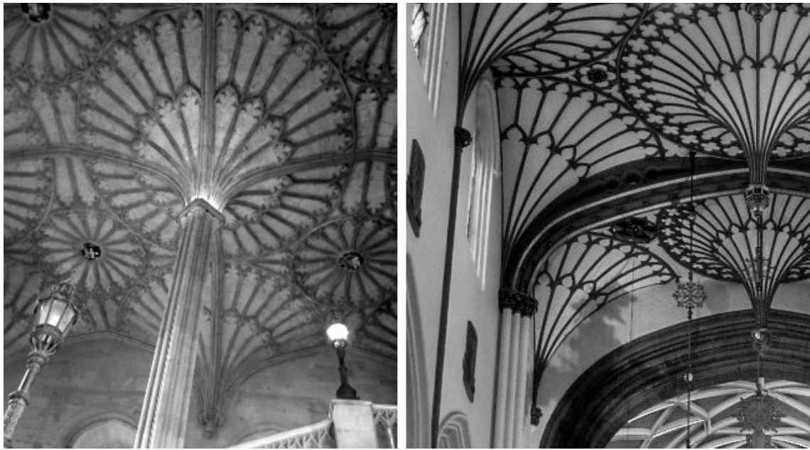
Figure 2.6: Composite Gothic pillar with fan vaulting, Christ Church Oxford (left) and St John's, Edinburgh (right). (Christ Church Photo: Katie Etherington, 2012)
