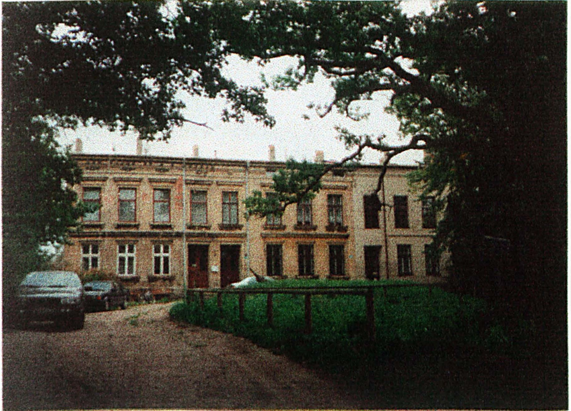
Blücherstraße 40 (formerly Alexandrinenstraße), Huhnhauser's house in Rostock. Second from left. September 1997.
