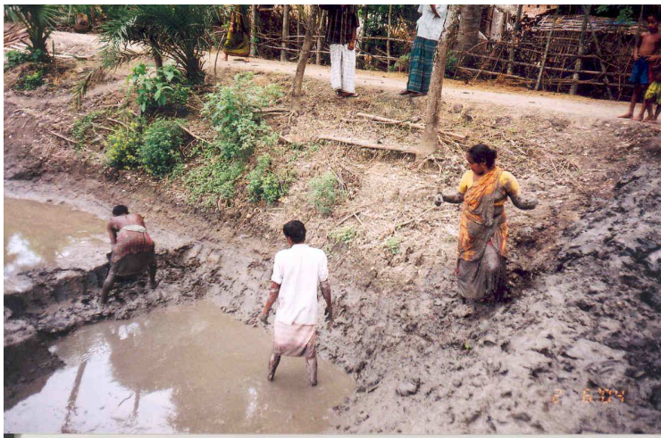
Photograph 3: Women involved in pond dike repairing
