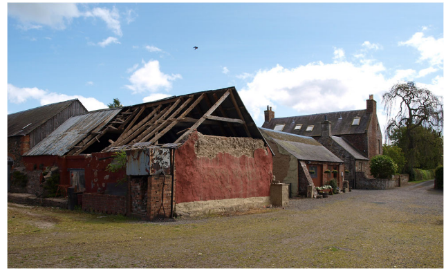
Fig. 2 Flatfield Steading, Perthshire. Later-eighteenth century group of farm buildings, two of which are of mudwall. These were cement-rendered in the 1970s to the detriment of the walling fabric
