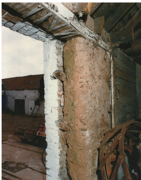
Fig. 6 Brick-faced claywall steading, Caldonshill Farm, Dumfries and Galloway, © Crown Copyright: RCAHMS. Licensor www.rcahms.gov.uk
