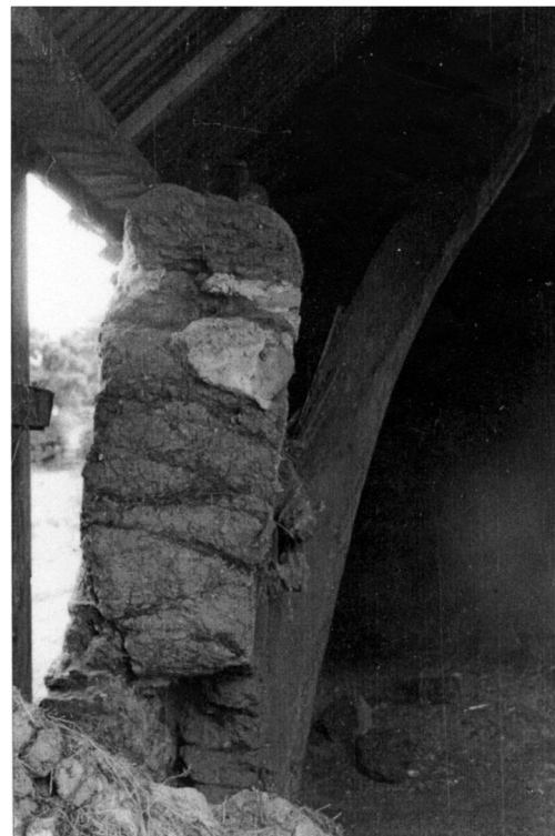
Fig. 3 Mudwall with straw layers included between lifts. Prior Linn farm, Canonbie, Dumfries and Galloway (taken by Werner Kissling in 1954 and held by the School of Scottish Studies Archive, University of Edinburgh)
