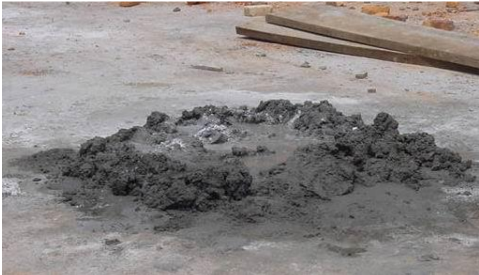
Plate 7-3: Some contractors ignore the rule by using conventional method
