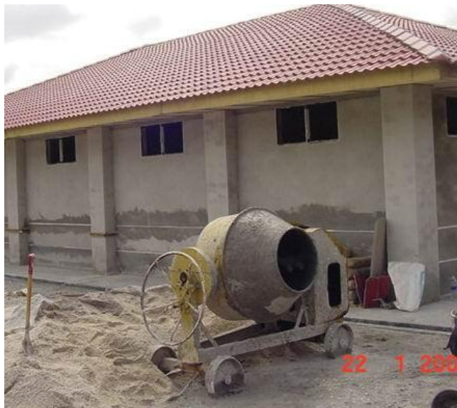
Plate 7-2: Simple building equipment is enough for this project
