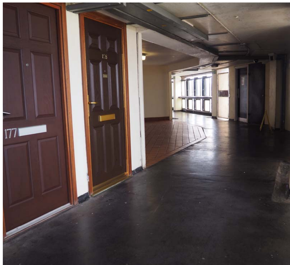
Figure 3. Cables Wynd House communal landing (photo by Respondent 3.8, reproduced with permission).
