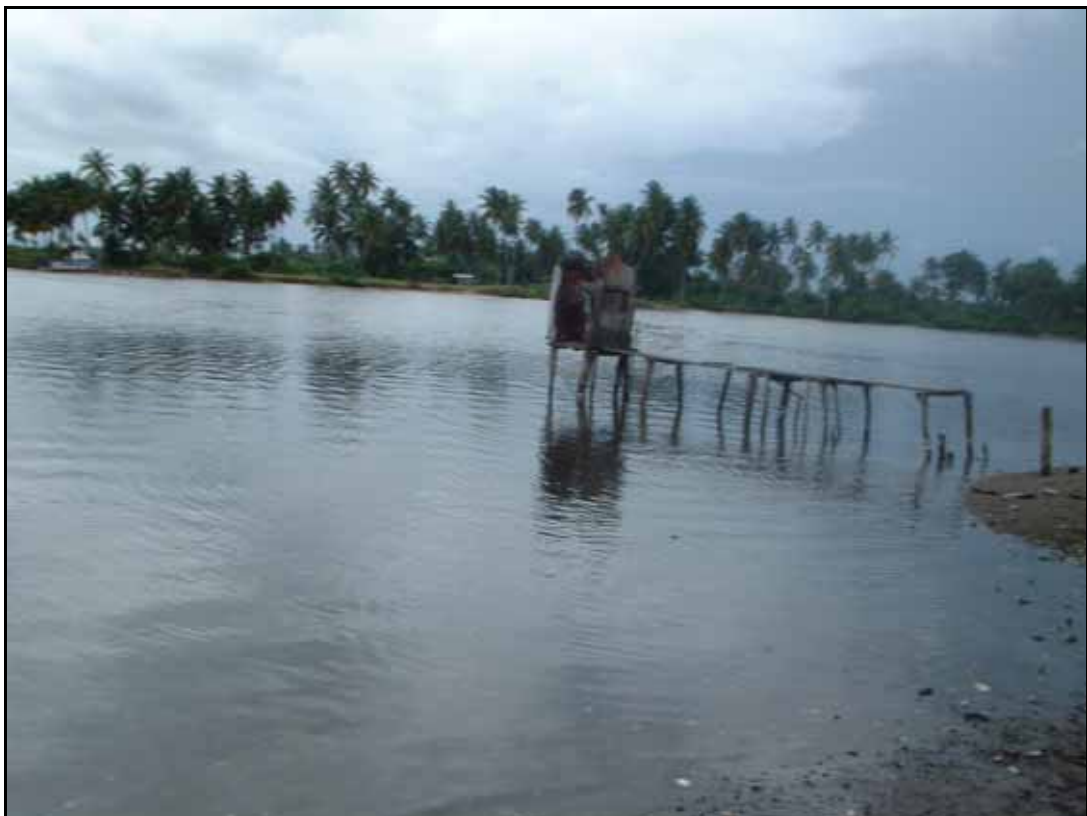
Figure 4.3: Toilet built over lagoon in Lagos state.
