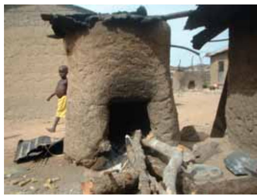
(b) Smoking kiln made of mud
