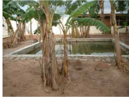
(b) Concrete fish pond in Niger state
