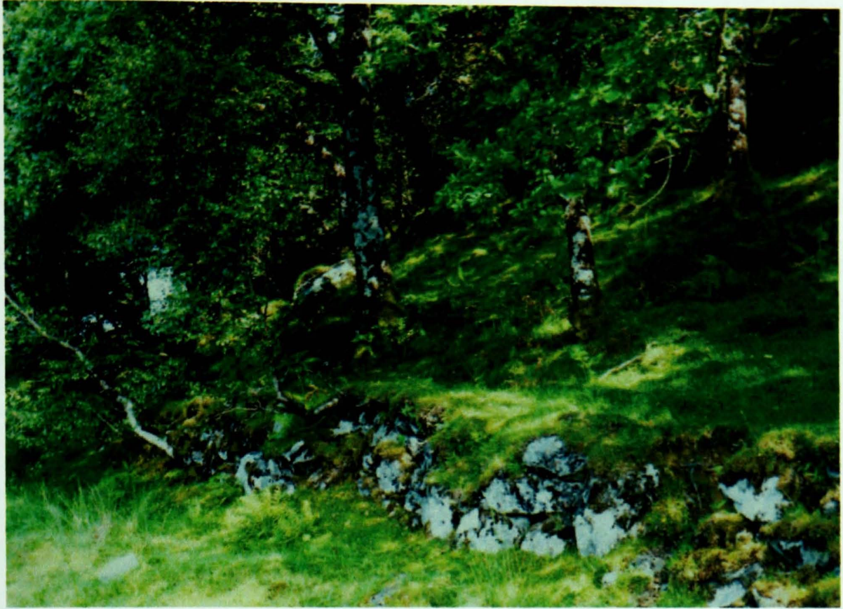
Figure 4-9 Boundary bank and wall, Lower Fernoch. When this was first made in 1721 it was expensive, but would provide a solid foundation for the protection of young coppice for the next 150 years.
