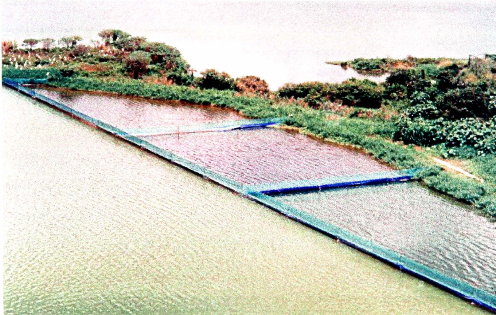
Figure 2.1: Overview of the experimental sub-areas isolated by PVC-reinforced sheets nearby the Northern Sewage Plant in the Bananal Branch, Lago Paranoá.
