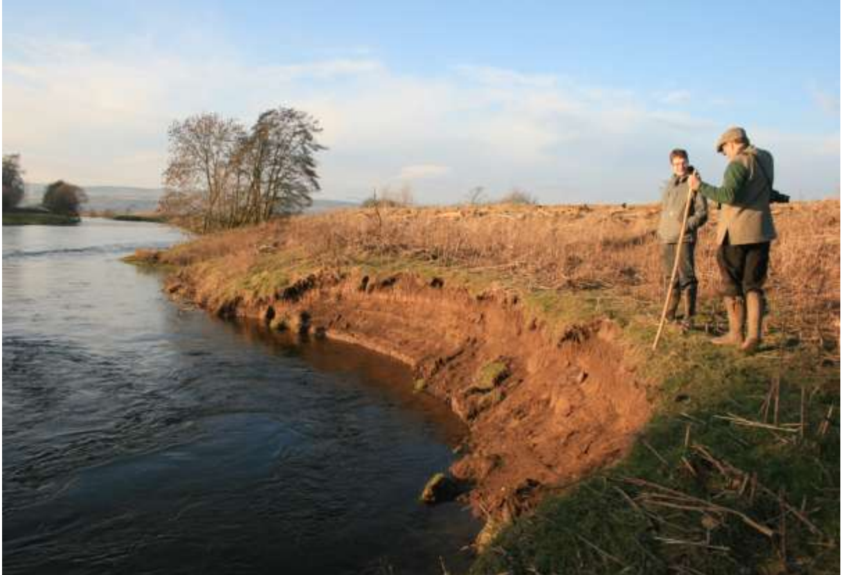
Fig. 7.10 The removal of riparian vegetation combined with seasonal floods, top-soil erosion and strong currents creates significant bank erosion, regardless of the presence of beavers (River Isla, March 2011 © Nigel Willby).
