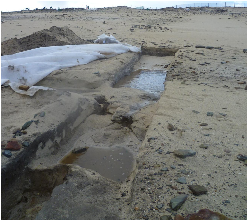
Figure 3.31: Soil test pit 5 during excavation.
