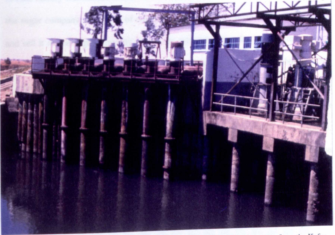
Figure 2.26 The water abstraction point at the end of the gravity canal diverting water from the Kafue River to Pumping Station 1, Nakambala Sugar Estate, Mazabuka.
