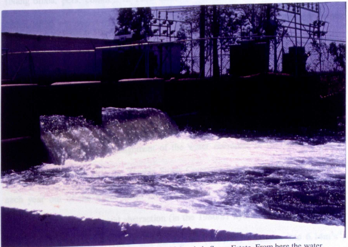
Figure 2.26 The water abstraction point at the end of the gravity canal diverting water from the Kafue River to Pumping Station 1, Nakambala Sugar Estate, Mazabuka.
