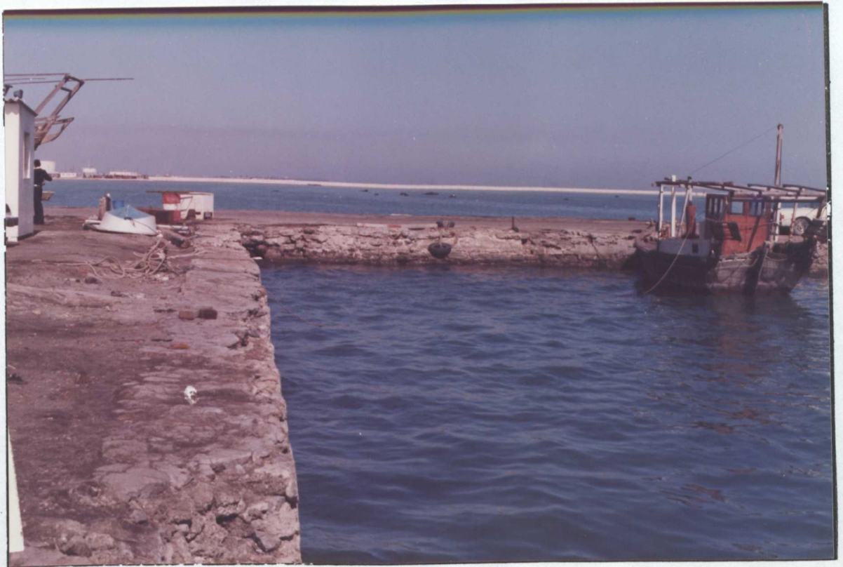
Figure: 2.16 Station 16 (Sitra jetty, Bander Al-Dar).
