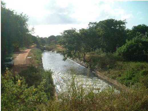
Plate 15: Irrigation channel, Mahweli H, Sri Lanka
