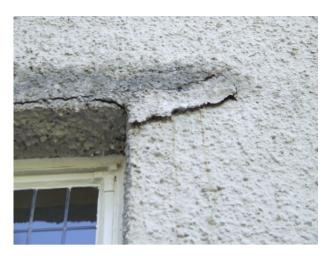
**Fig. 7.** Example of the cracking in the Portland Cement render of the Hill House, Helensburgh. Cracking such as this allows water ingress that threatens the historic Macintosh-Macdonald designed interior decoration and furniture (Photograph: John Hughes).
