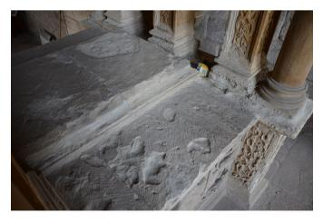
**Fig. 5.** Decay on the top of the tomb at the Skelmorlie Aisle, Largs. Here the dense fine-grained sandstone is suffering from cratering and powdering. At the centre top right of the image, an environmental logging device can be seen attached to the structure, recording conditions of Temperature and Relative Humidity near to where the damage is occurring (Photograph: Maureen Young, Historic Environment Scotland).
