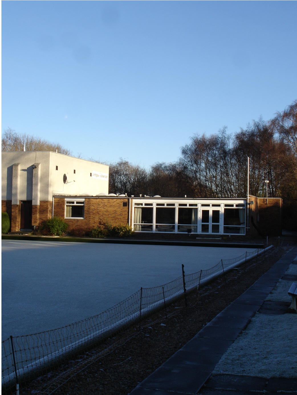
Figure 105 : Linlithgow Tennis Club – View to the Clubhouse across the Bowling Green
