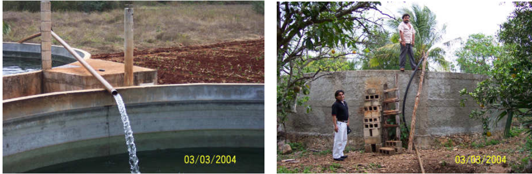
Figure 3.11 Round tanks used by the social sector in Yucatan, Mexico.
