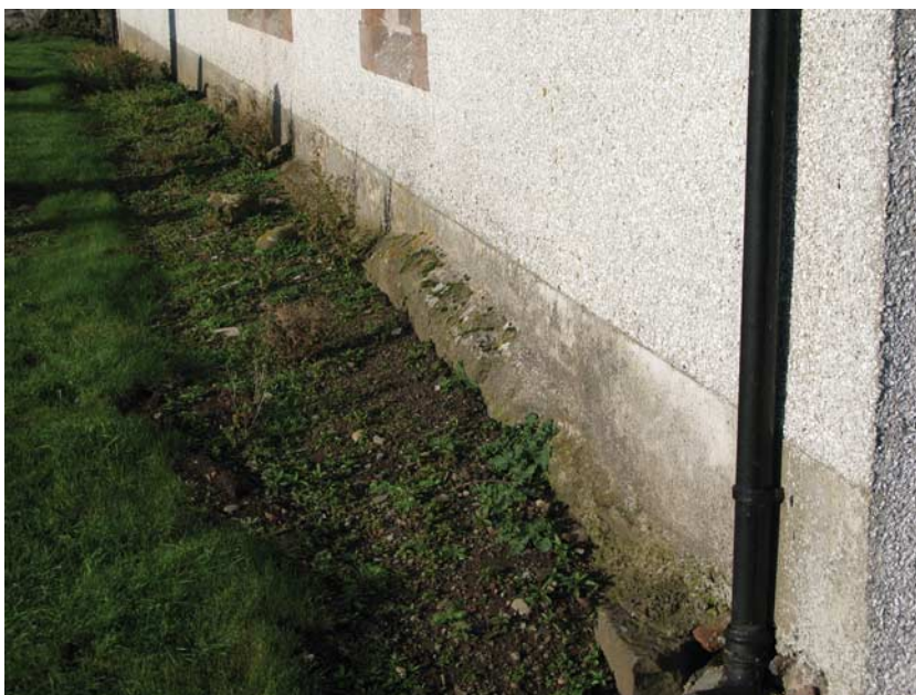
Fig 6. Madderty church, showing the earlier foundations projecting below the south wall
