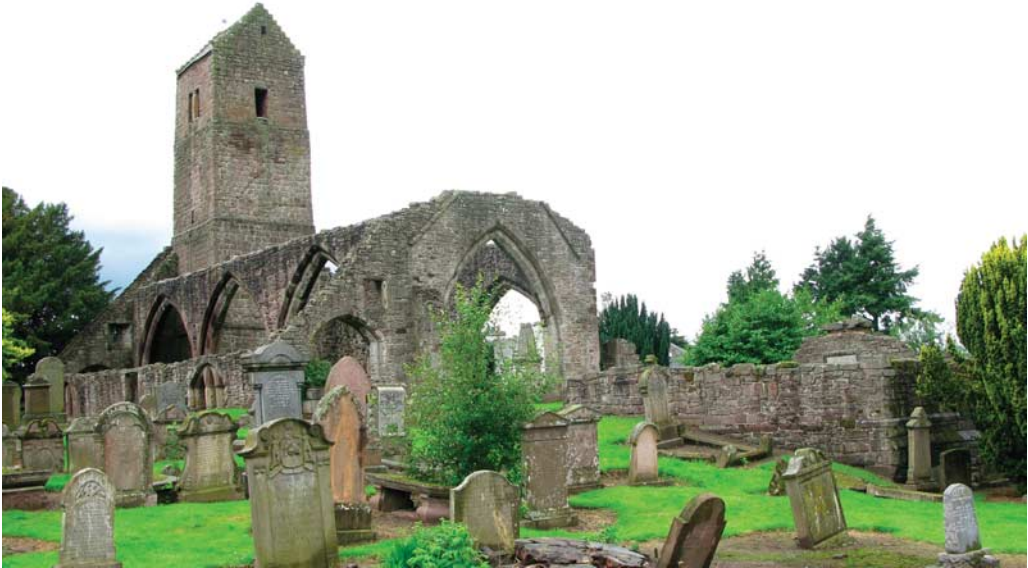
Fig 17. Muthill church from the south east. This was one of the most ambitious non-cathedral parish churches in the study area; the nave aisles were a secondary addition to a three-compartment plan
