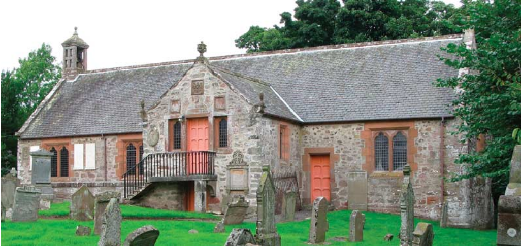
Fig 16. Forgandenny church from the south. The aisle projecting from the south flank may have originated as the chapel of St Katherine, which was founded in 1494, but it later became the aisle of the Ruthven of Freeland family
