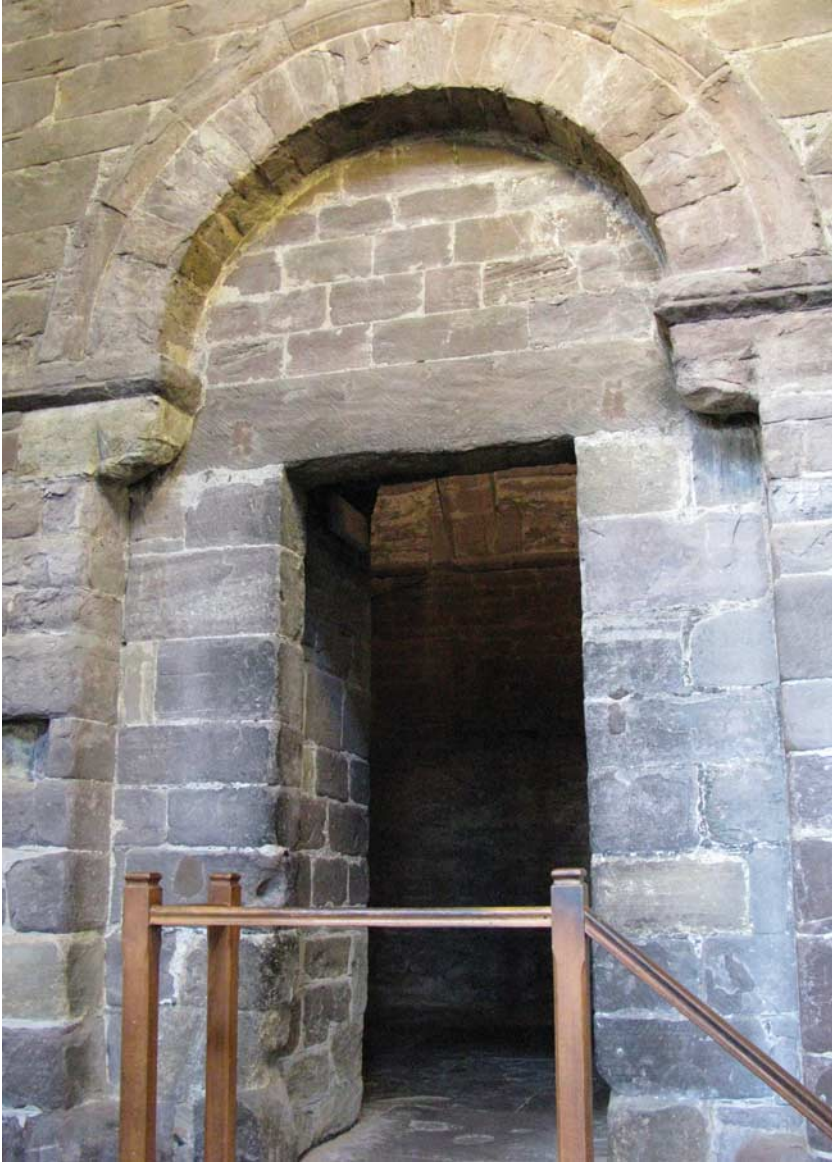
Fig 24. Dunblane cathedral: the doorway in the north face of the tower
