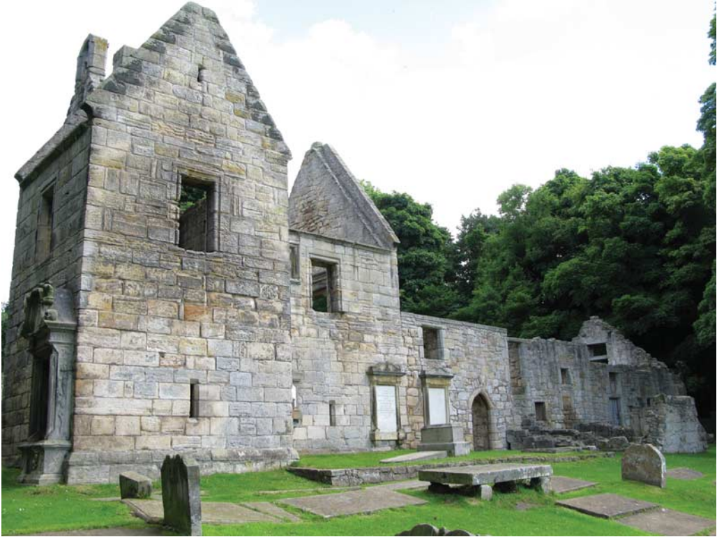
Fig 4. Dalgety church from the south west. The enormous two-storeyed laird's aisle of the first earl of Dunfermline extends from the west end of the rectangular medieval church, while the fragments of another laird's aisle project from the south flank
