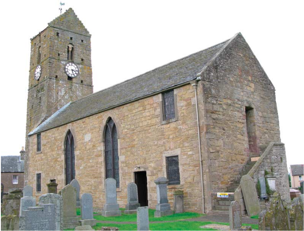
Fig 2. Dunning church from the south east. The structural distinction between chancel and nave was partly suppressed when the south wall was rebuilt in 1810
