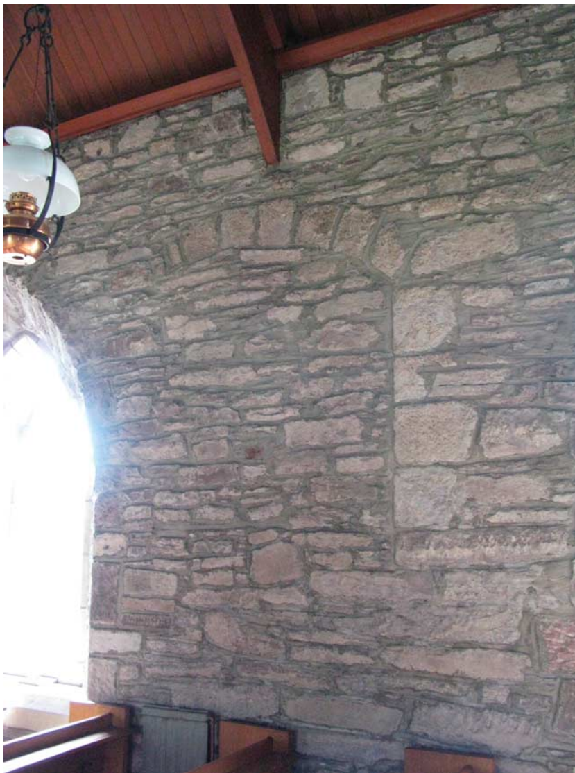
Fig 7. Fowlis Wester church, showing traces of an earlier window rear arch in the south wall
