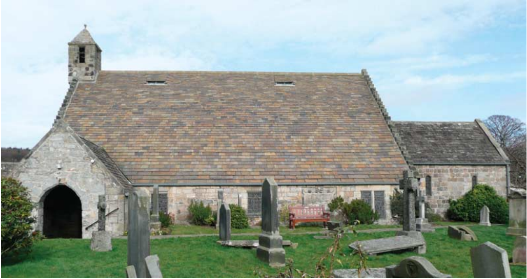
Fig 19. Aberdour church from the south. The later south aisle is covered by a continuation of the nave roof
