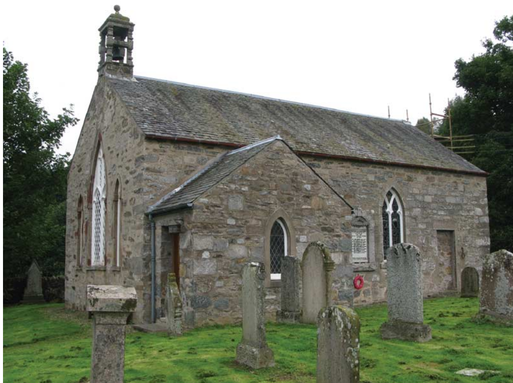
Fig 15. Dowally church from the south east. This church, which has been truncated, was under construction for Bishop George Brown in 1510
