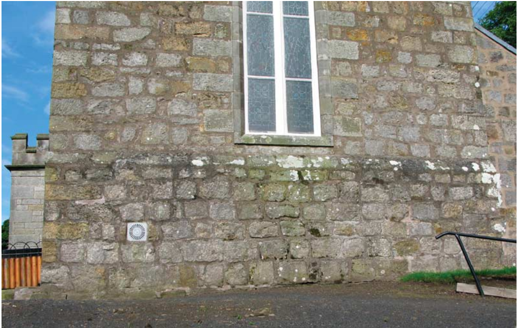
Fig 9. Aughtertool church, showing the earlier masonry and base course along the east wall
