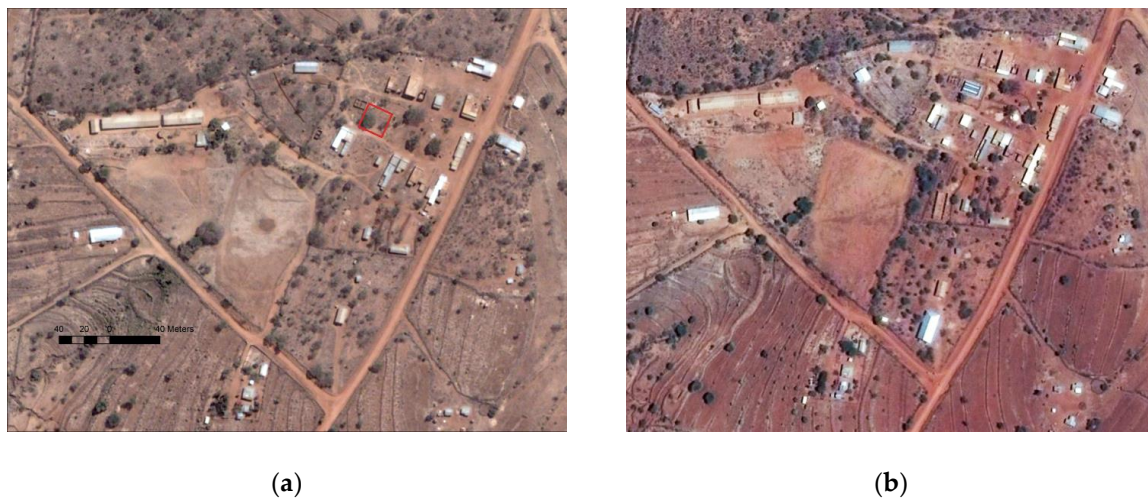
Figure 4. (a) Kitonyoni trading centre in 2012, prior to energy access intervention. Red square is the (future) location of the solar power plant; (b) Kitonyoni trading centre in October 2013, 1 year after the installation of the solar mini-grid.
