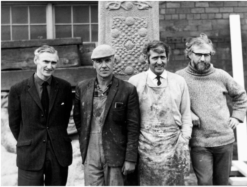
Figure 5. Engineer John Scott who led the SJC project for Exposagg Ltd, conservator Tam Day, foreman plasterer Jackie Drysdale, and artist John Lawrie stand in front of the freshly cast concrete in Borthwick's Yard, Edinburgh, before it journeys to Iona. Photograph by Arthur MacGregor, reproduced with permission from HES.
