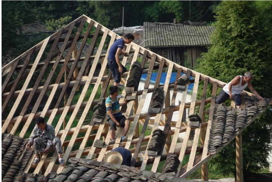
Figure 7: Social workers and villagers doing tiling
