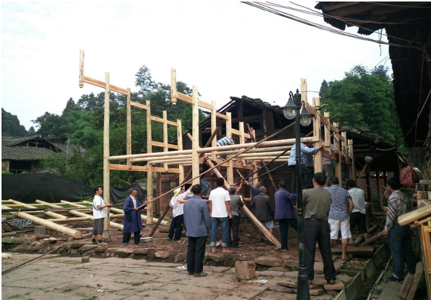
Figure 6: Villager setting up the frame of building collectively
