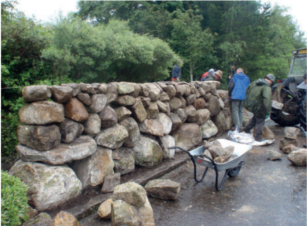
Dry-stone wall restoration work. Credit: Mourne Heritage Trust
