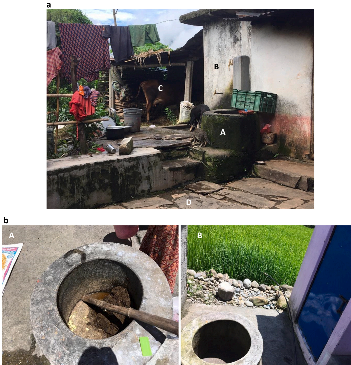
Fig. 5. a: TLAD in a rural household in Nepal. The components of the system are as follows; Cow dung and food waste inlet (A) Toilet (B) Animal holding close to house and digester (C) the main TLAD digester dome is situated underground (D). b: Two cow dung and food waste inlets. (A) shows the inlet with cow dung prior to users mixing with water and moving a stone that blocks the inlet pipe to the digester so the liquid mix can fall via gravity into the digester, (B) shows an empty cow dung and food waste inlet next to the toilet (blue door) and rice field behind the house, the slurry exits the digester and flows freely into the rice fields or can be composted first. (For interpretation of the references to colour in this figure legend, the reader is referred to the web version of this article.)
