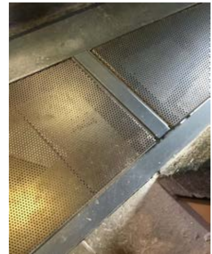
Perforated decking can be difficult to cross.
