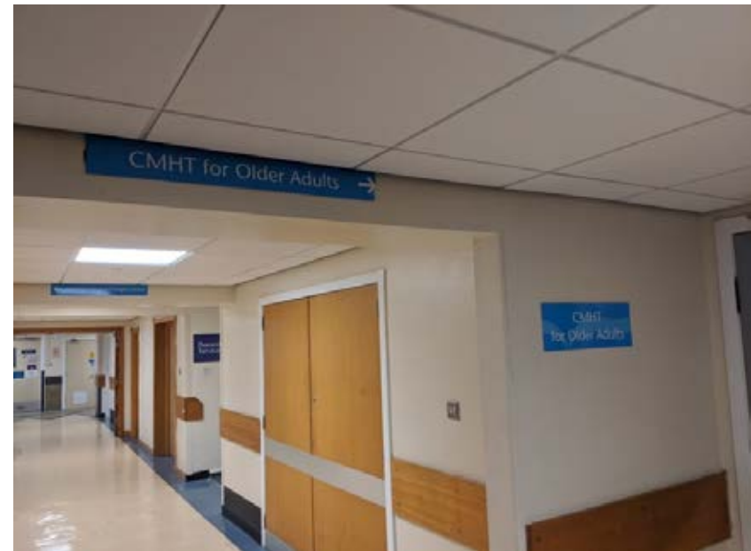
Good practice signage was often undermined by being applied in a patchy or inconsistent manner. Colour coding that was not explained can cause confusion.
