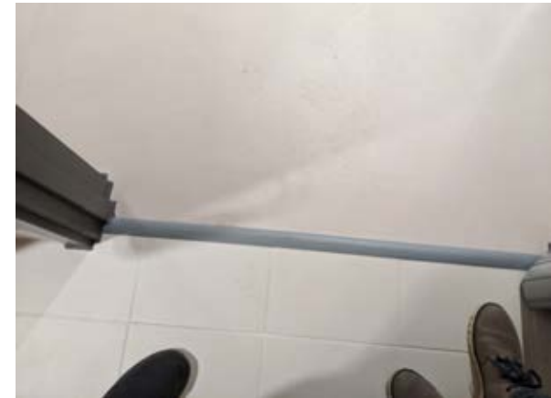
Overall, the design of the Bellfield Centre is positive with only a handful of items for improvement. E.g. contrasting threshold strips
