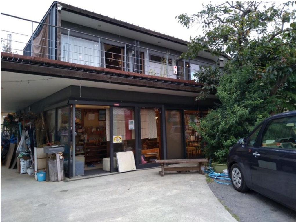
Photo 4. Aoi Care shared residential unit.
