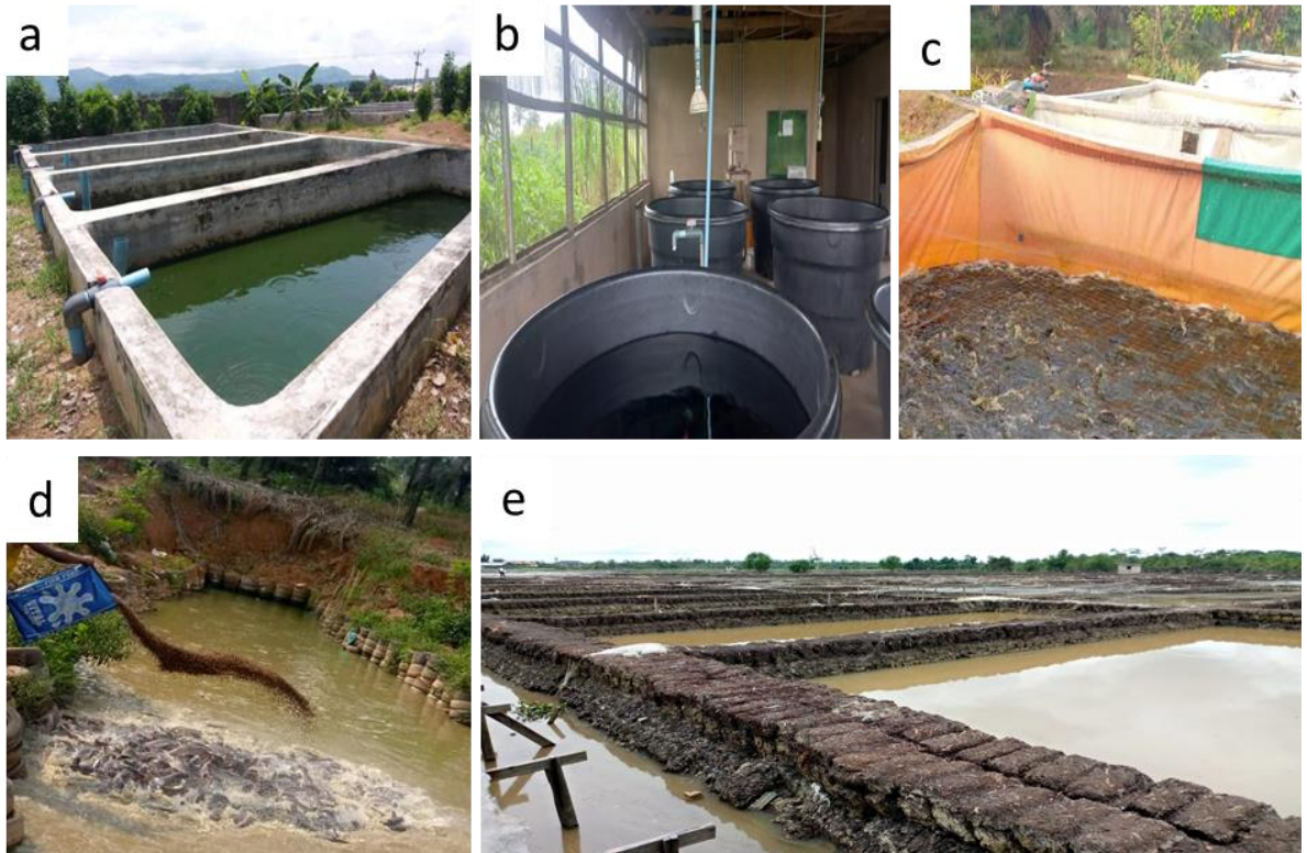
Figure 2.6: Examples of aquaculture facilities commonly used in Nigeria. Concrete pond sitting on ground level (a), layout of indoor plastic tanks (b), improvised facility using tarpaulin and wooden frames (c), Fishpond wall reinforced with sand-filled tyres (d) and a cluster of earthen ponds with water canals (e).
