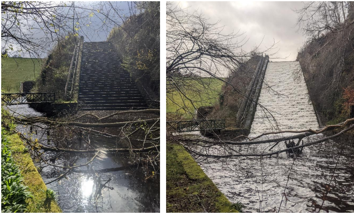
Figure 1.4: Example of varying flow regimes from a hydroelectric dam with stepped spillway. With the spillway active, the downstream environment becomes more oxygenated through turbulence, despite only a modest rise in river level. Dam located on Edgelaw Reservoir, Midlothian. Images taken by R. Steenson (2021).
