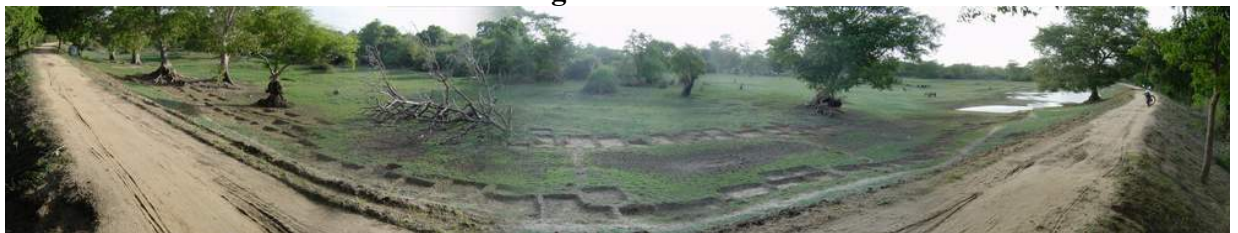
19 October 01 – Showing areas excavated for bund repairs
