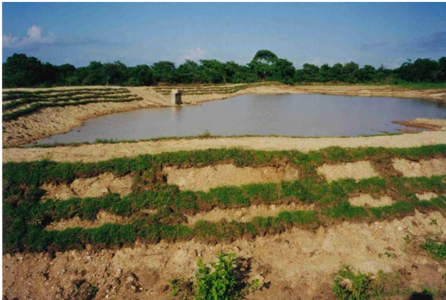
Plate 2.3 Keeriyagahawewa; a radial tank in the Anamaduwa research area, partially filled, two months after being fully renovated in September 1999. Works included, full de-silting, surplus weir, sluice and bund repairs.
